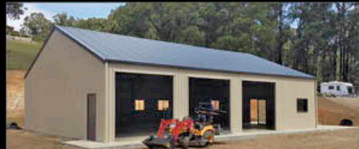
65) Small Machinery Shed 12m x 16m x 3.8m with 22° Roof Paperbark® walls | Basil® doors & trim
