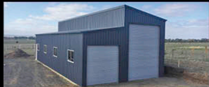
67) Skillion Roof 4m x 16m x 4.3m with 4m Lean-to (1.3m drop) Deep Ocean® walls | Evening Haze® doors
